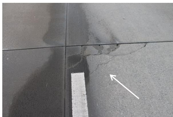
Figure 2: Close-up view of a joint cross with water outlet from the joints, cracks around the cross and partially collapse and subsidence of the concrete (s. arrow).
