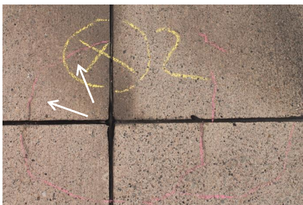
Figure 3: Extraction point of the core 2, which is located in the area of a longitudinal joint on a crack present there (s arrows).
