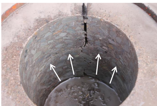
Figure 5: Borehole of the core 2. Here it can be clearly seen that, starting from the base of the saw cut, a surface-parallel crack has developed (s. arrows).
