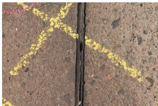
Figure 4. Close-up of a sealing gasket in the joint. It can be seen that the seal is perforated. Water penetrates through the hole.
