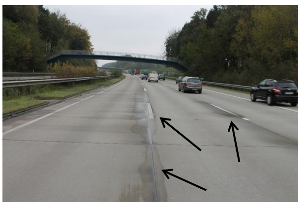
Figure 1: Concrete roadway of the Bundesautobahn A1; here the water comes out of the longitudinal joints (s. arrows).
