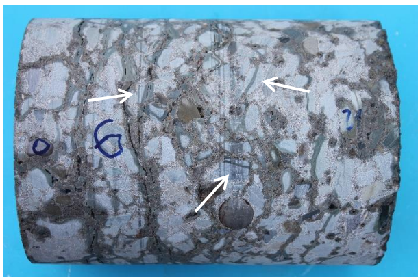
Figure 7: Mantle surface of the structural concrete of core 6, dipped in water for visualization of cracks present in concrete, during its advanced drying. The concrete is interspersed with AKR-typical cracks. Some of the cracks run through the coarse aggregates (see arrows).
